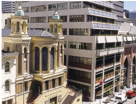
Aspect San Francisco's superb downtown location
